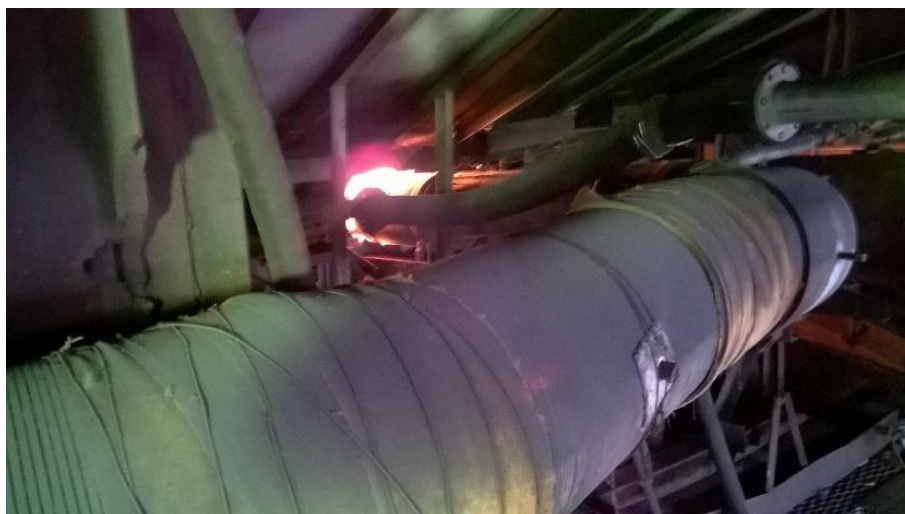
Figure 5. Photo of the air duct for feeding husks into the rotary kiln furnace.
