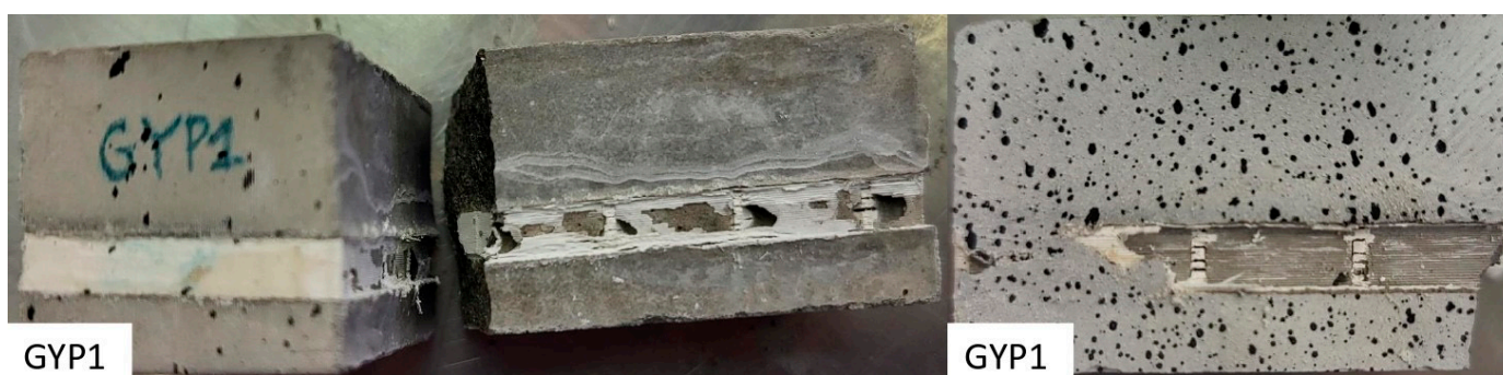
Figure 10. Formation of holes in the GYP material reinforced concrete with white precipitation.
