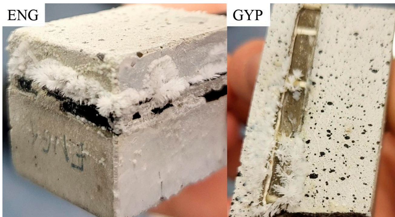
Figure 17. Occurrence of white crystals on the reinforced concrete beams kept underwater for four weeks.
