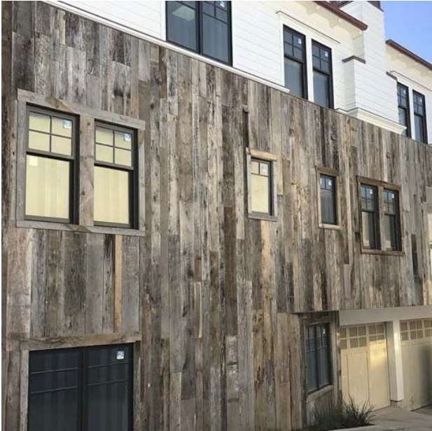
Fig. 3.27 - Example of Reusing Wooden Planks in Facade Finishing [62]
