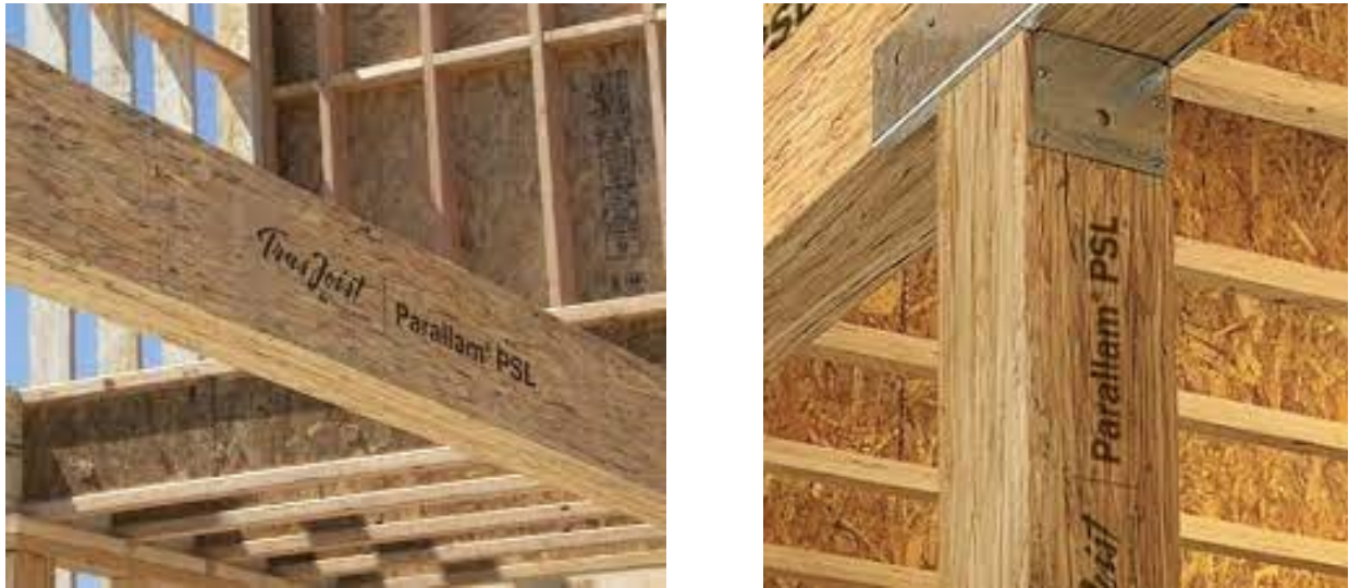
Fig. 3.8 - Parallel Strand Lumber (PSL)
