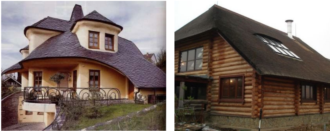
Fig. 3.26 - Photos of Modern Individual Houses Made from Locally Sourced Materials (cob - clay and straw mixture, timber walls, thatched roof) [60, 61]
