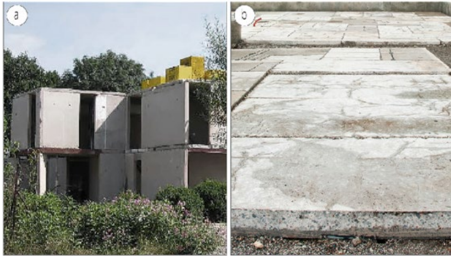
Fig. 3.24 - Concrete Upcycling (Reuse of Wall Panels in Road Pavement) [57]
