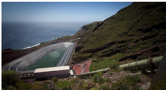
Figure 3 – The lower reservoir and hydropower station at the Gorona power station on El Hierro Island (3)
