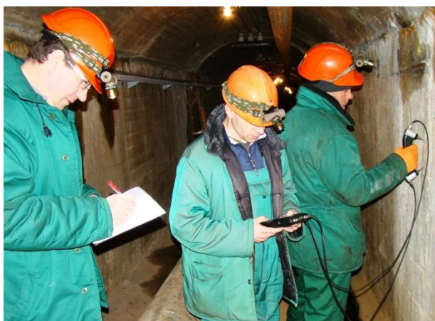
Figure 9. Strength of concrete determination with ultrasonic method.
