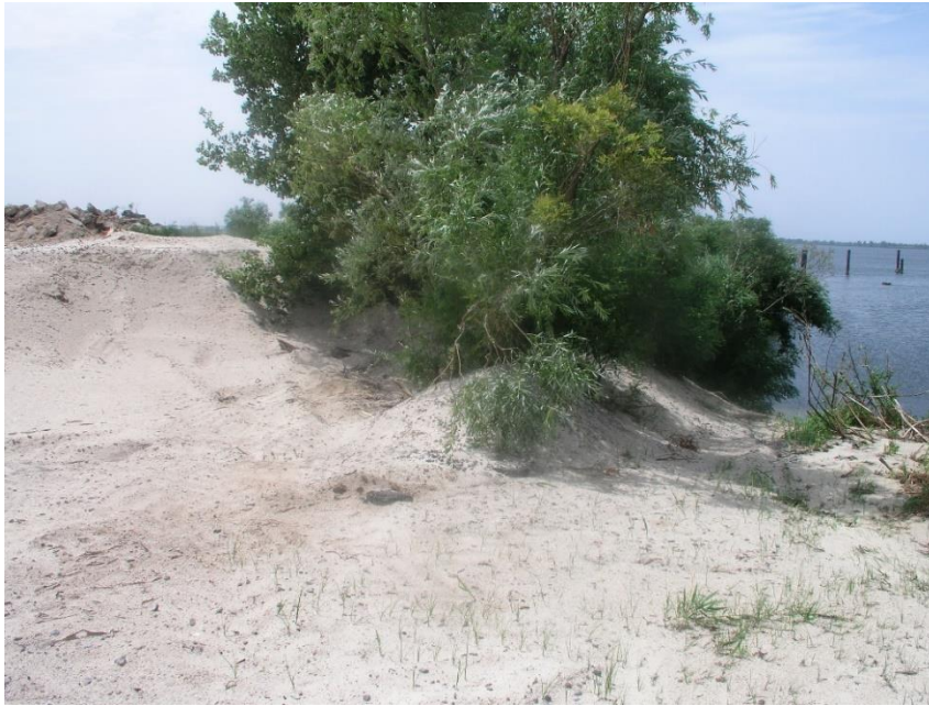
Fig. 4. Reworking of the coastal slope of the cooling pond dam from the side of the Kakhovka Reservoir (photo 2010)
