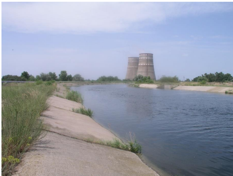
Fig. 1. The tail-water channel from the cooling towers on the dam of the Zaporizhzhia NPP cooling pond (photo 2010)
