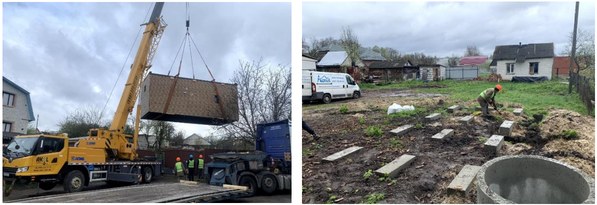
Fig. 2. Installation process of single-family modular prefab
