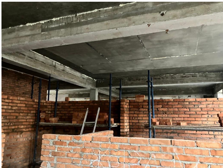
Fig. 2.1 Restoration of damaged residential building in Pokrovsk, Kherson Region
