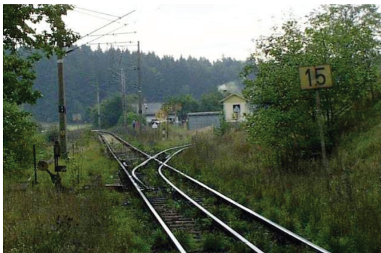
Fig. 1 Three-rail track near the station
