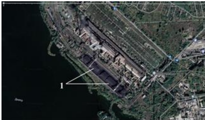
Figure 1. Prydniprovskaya TPS: 1 – a pile of coal (Google Image, 2022).
