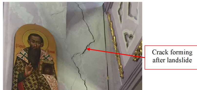
Figure 2. Deformations of the St. Illia Church.
