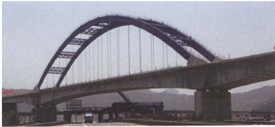
(a) Kuyang Bridge
