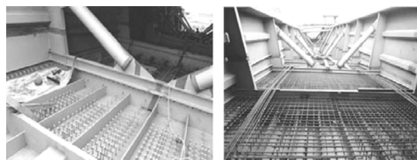
Fig. 14. The bottom concrete plate connected with steel by means of shear stud connectors [8]
