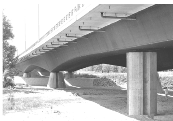
Fig. 7. The highway bridge over the Ostravice River in Ostrava, Czech Republic
