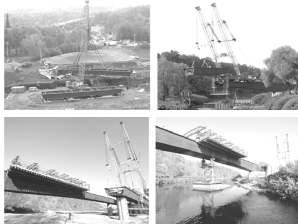
Fig. 10. The bridge construction stages [4, 5]
