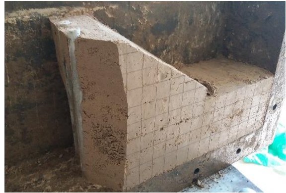
Fig. 5. Appearance of the soil cement elements in the bank body after the test
