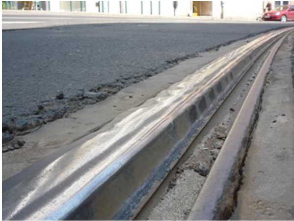
Fig. 3. Mixed type rail wears in R = 63 m radius curve
