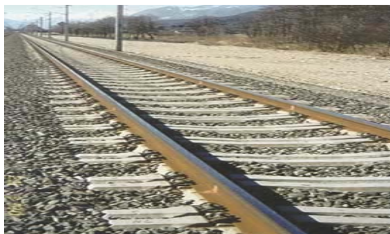
Figure 5 A track on concrete framed sleepers on the Turin Line (Italy)
